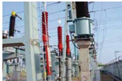
110kV dry style termination applied in Zhuhai
